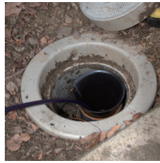
Insert Sleeve in the cleanout
