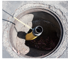
Tiger tail used on a manhole
